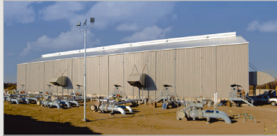
Joliet Compressor Station
